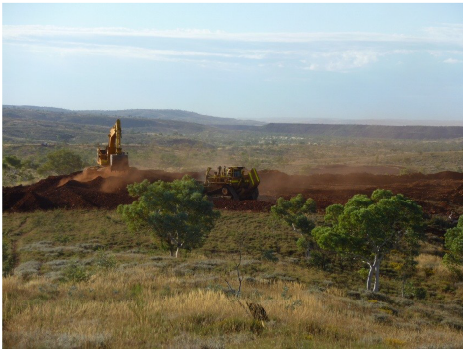
Cut and fill operations in the ROM area
