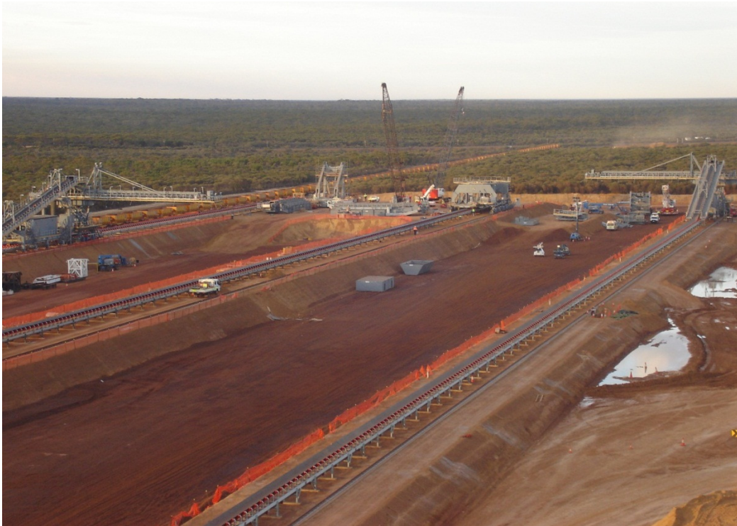
Stockyard earthworks and machine assembly at Carina Ore Handling Plant
