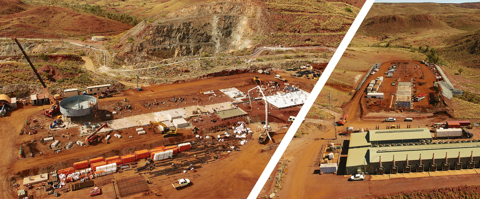
Images: Construction progressing on beneficiation and power plants
