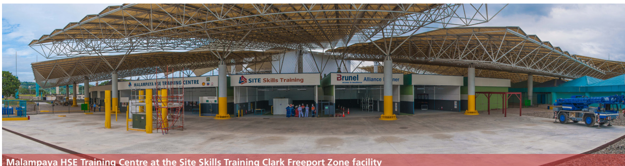
Malampaya HSE Training Centre at the Site Skills Training Clark Freeport Zone facility
