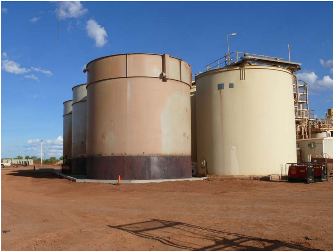
Figure 2: Installation of three additional leach tanks
