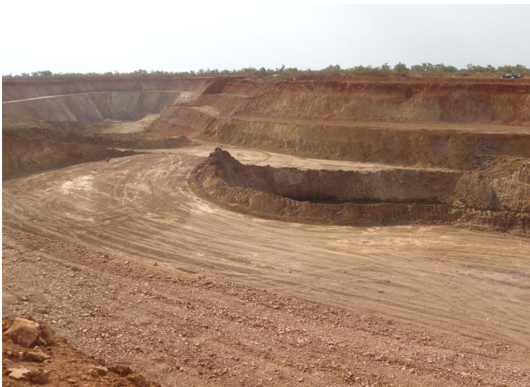
Sandpiper Pit looking North West - 350mRI in West portion and 360mRI in central saddle area.
