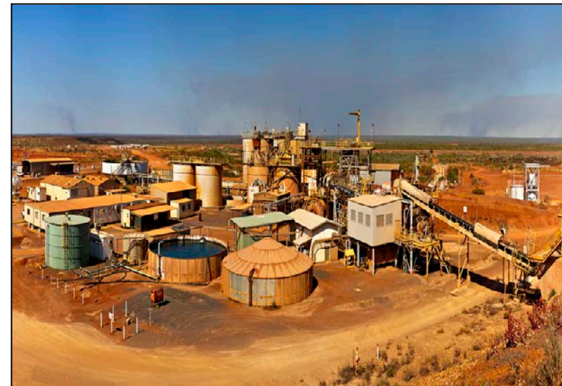
CTP Processing Facility
