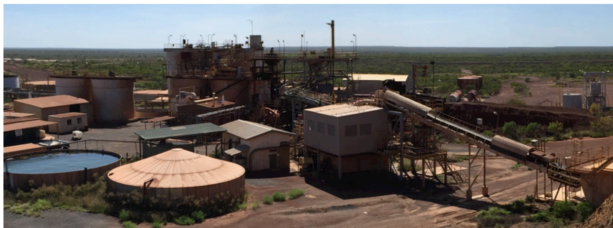
[ CTP Processing Facility ]
