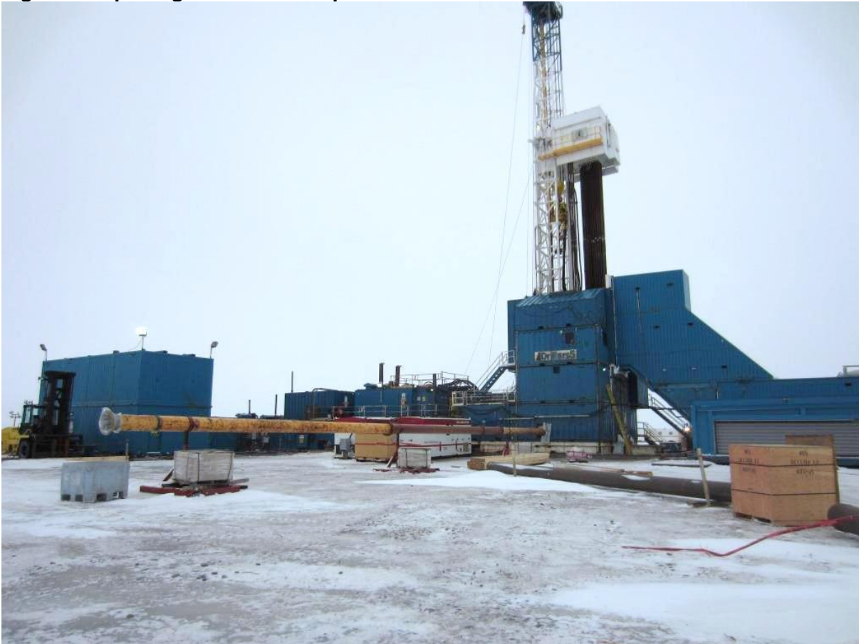
Fig 1. Kuukpik Rig Just Prior to Spud
