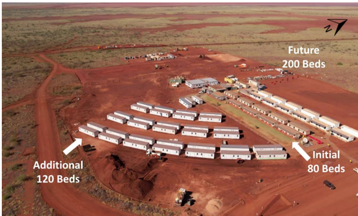
Figure 4: Mardie Accommodation Facilities Expansion
