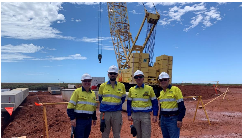
Figure 1: Construction underway at Pond 0
