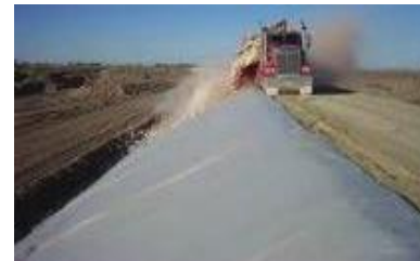
POND 5 EMBANKMENT TRIAL
