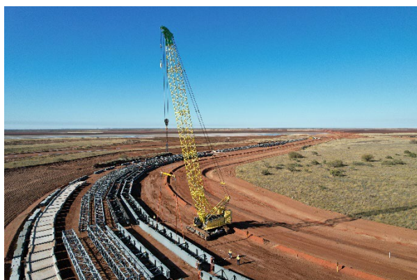
Figure 3: Jetty lay down area
