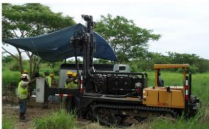
Sonic drill rig
