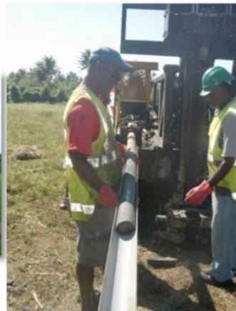
Sonic drill rig 'core'
