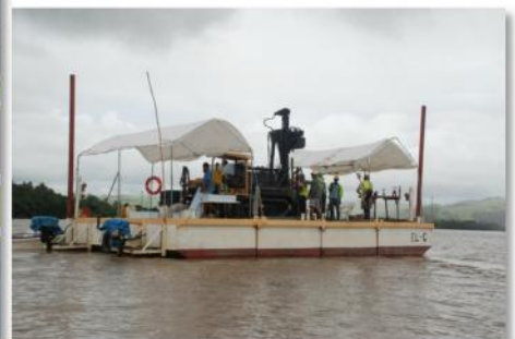
Drilling in the river
