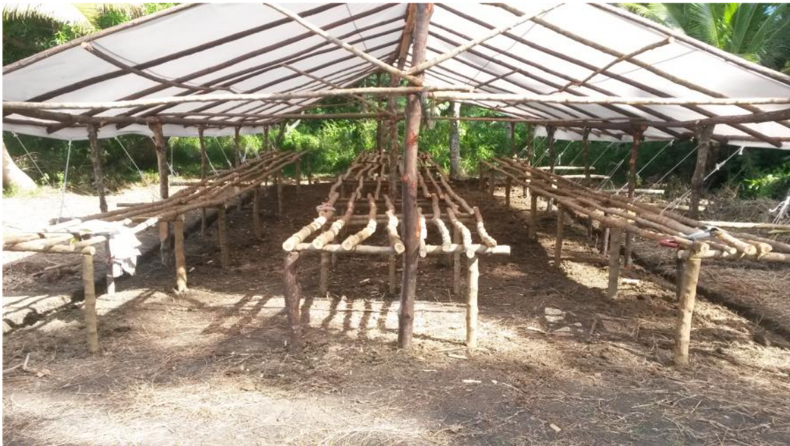
Plate 1 - Diamond drill core logging building with bench space to layout entire drill holes
