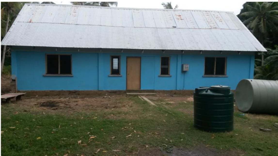
Plate 2 - Office and accommodation building with water storage tanks ready for installation
