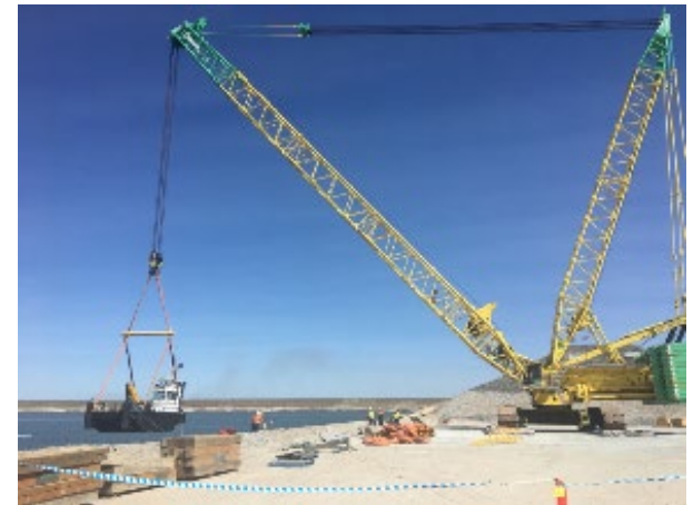
Workboat Ginga being placed into the Tailings Storage Facility
