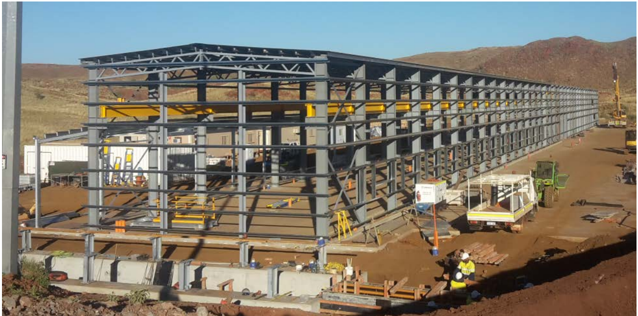
Progress of Engine Hall Construction – Wodgina Lithium Project
