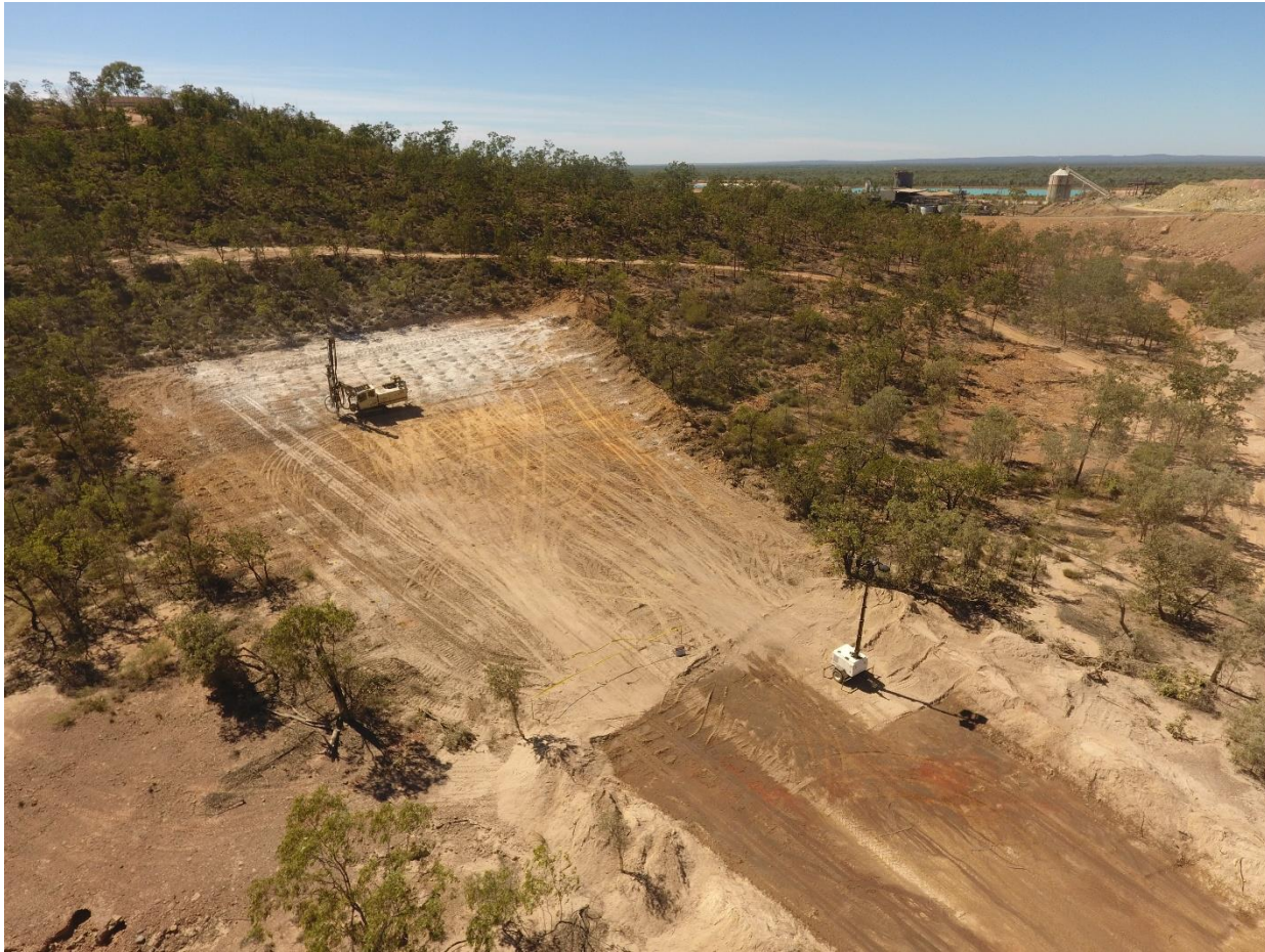
Figure 2 Blast hole pattern being drilled at Far West Portal
