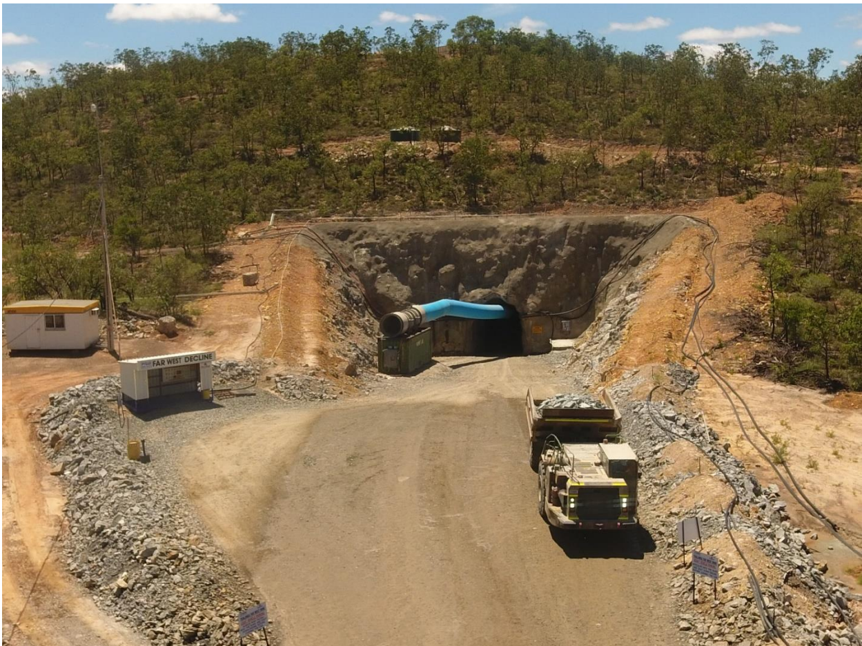
Figure 1 Ore being hauled from Far West decline
