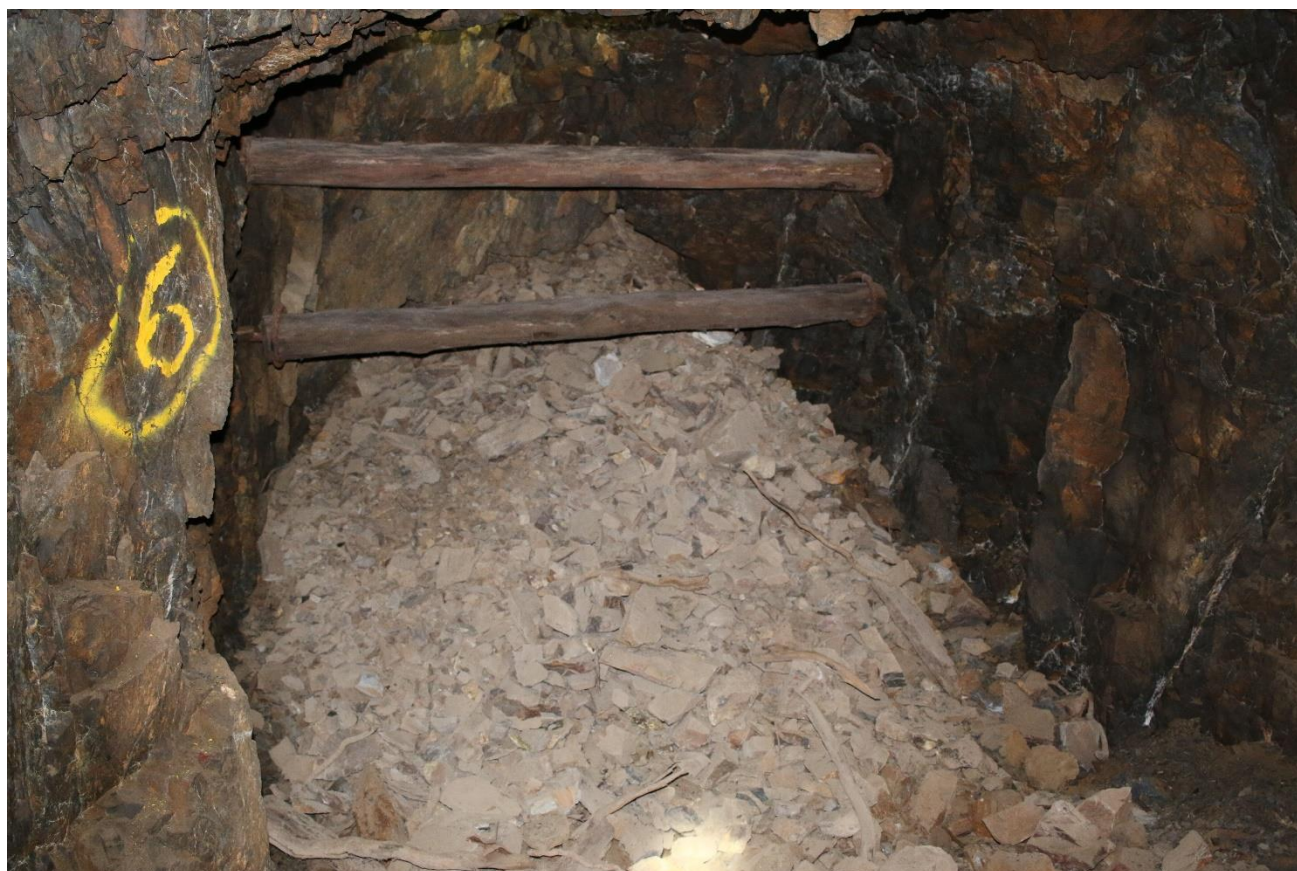
Figure 5 Draw Point 3 (DP3) 1700 Level
