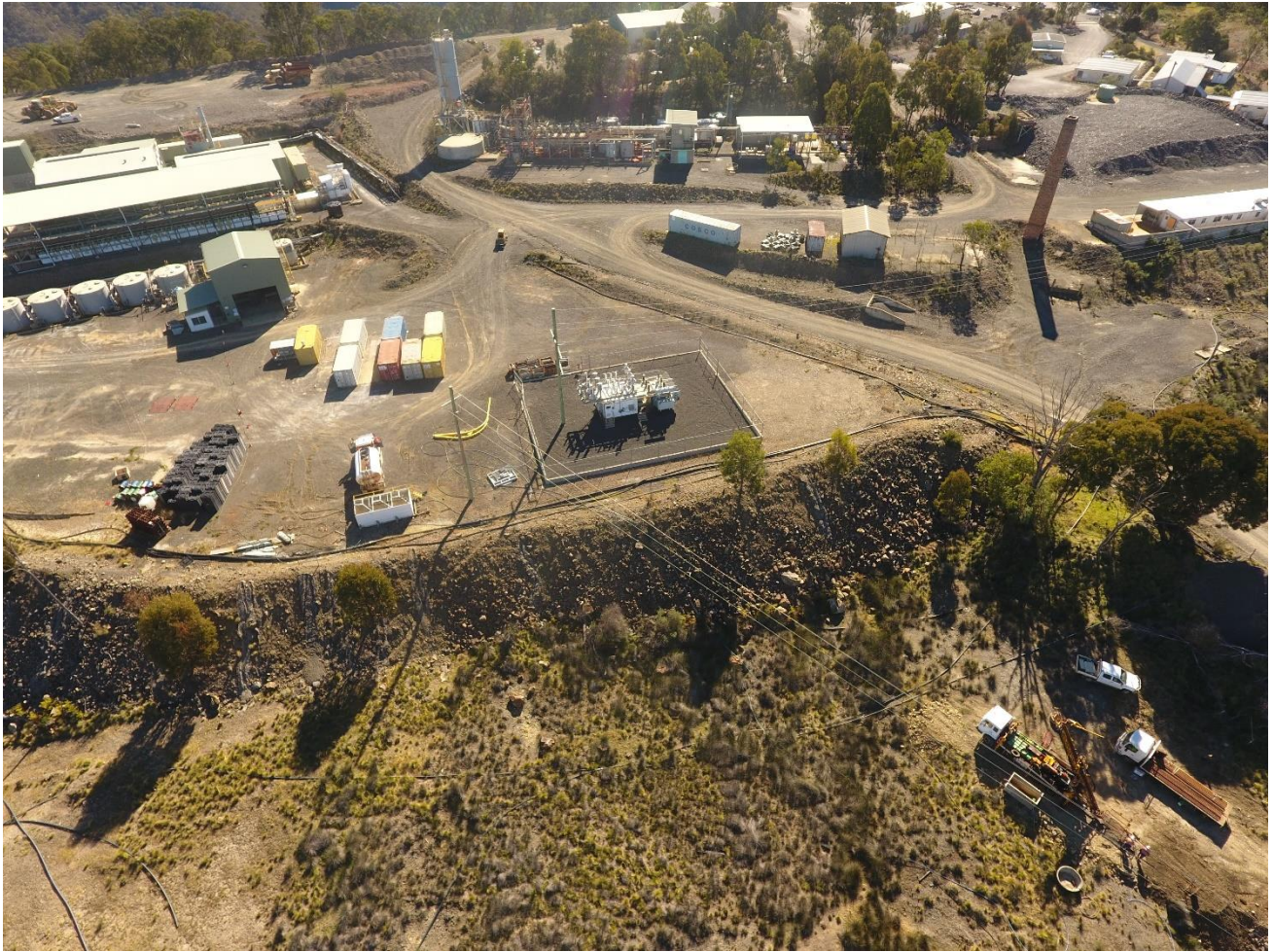
Figure 2 Drilling commencing at Eleanora Uppers
