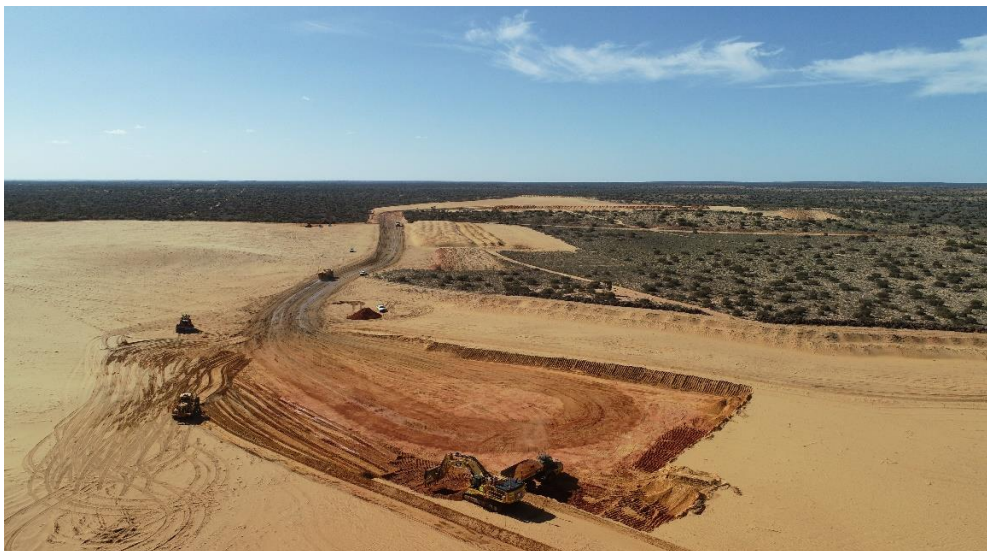
Figure 1 Early works at Mulga Rock – excavation of the Ambassador North pit
