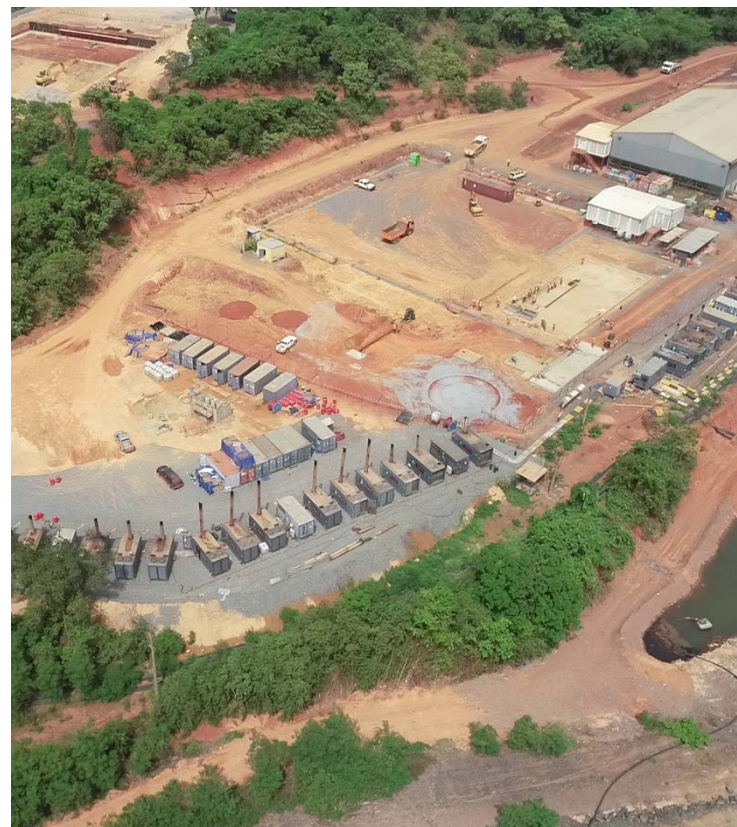
Photo: Progress at new Syama Power Plant
