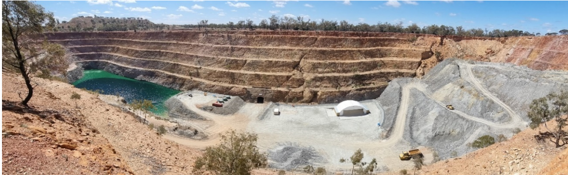
Figure 1 – Surface facilities and portal for Avoca Tank access decline.
