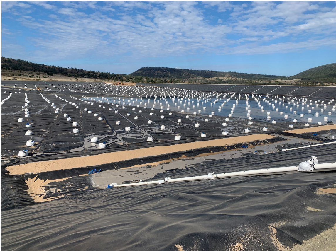
Figure 3 – First tailings being deposited into Tailings Storage Facility No.2
