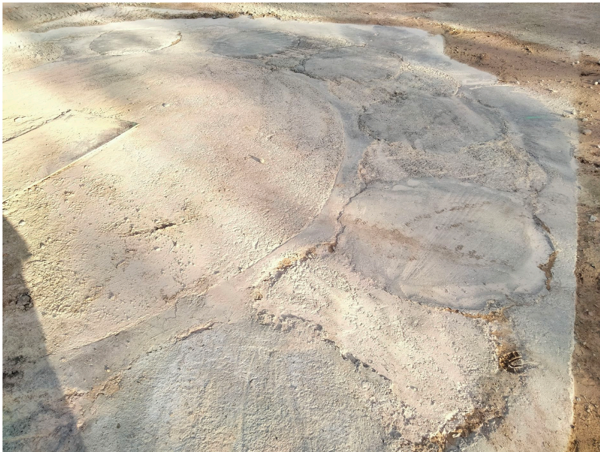
Figure 5 – Completed pilings at Budgerygar
