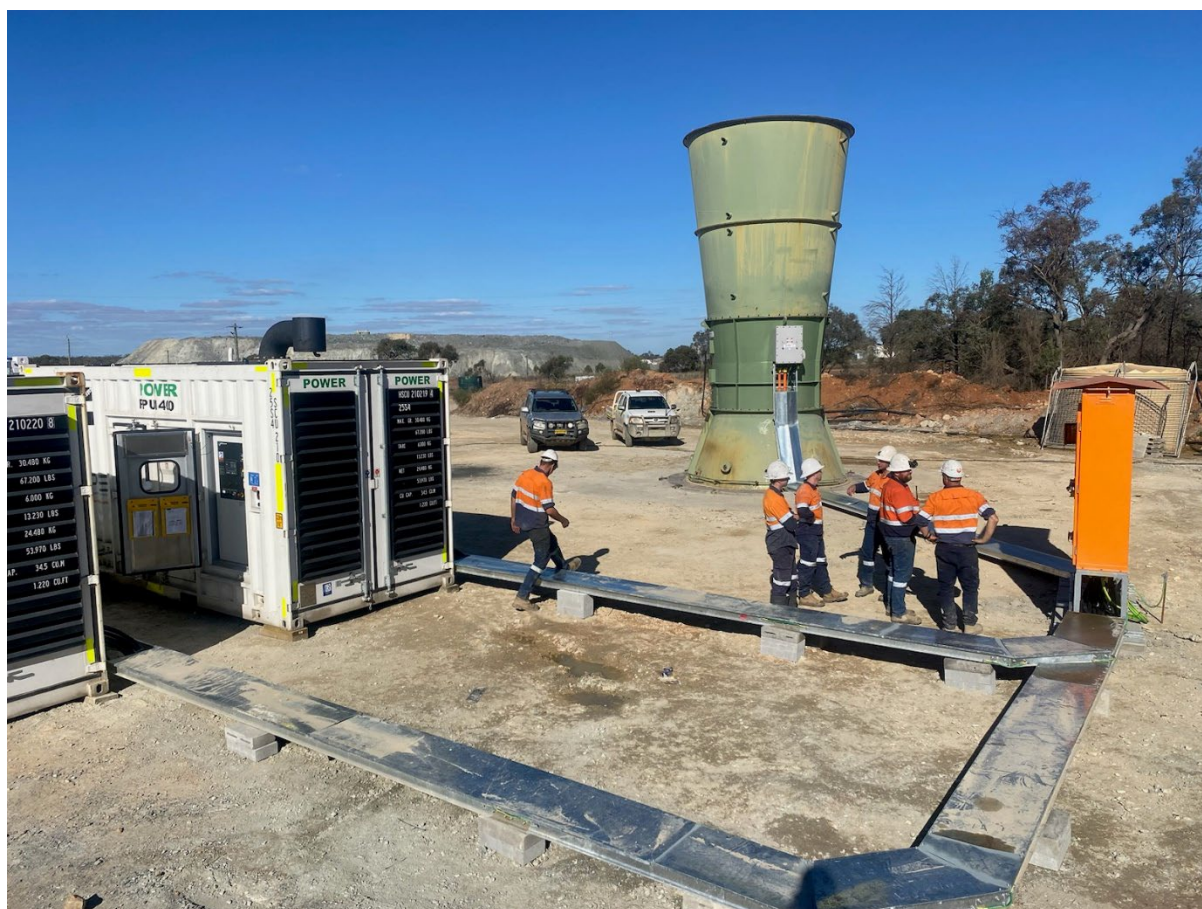
Figure 2 – Completed Budgerygar ventilation shaft
