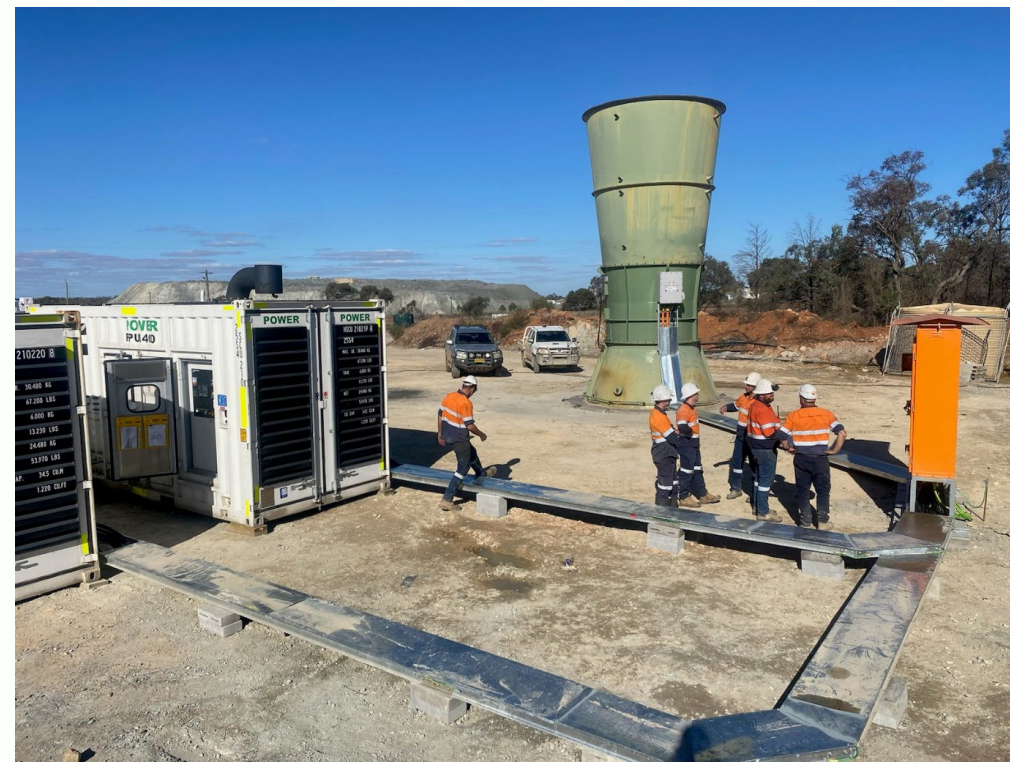
Completed Budgerygar vent shaft at Tritton
