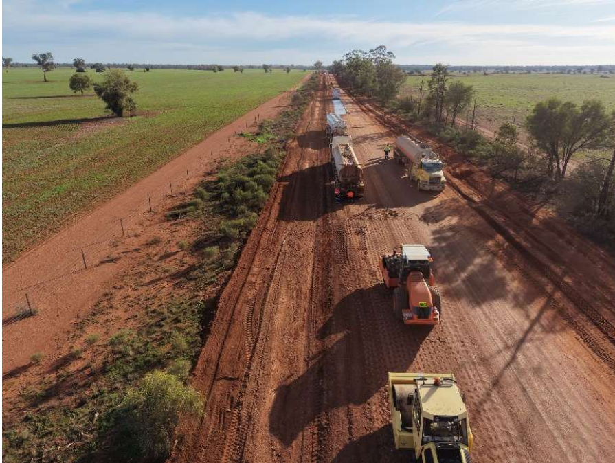
Figure 3: Constellation haul road construction
