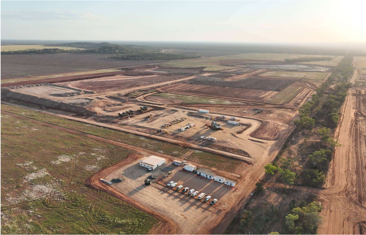
Site construction underway
