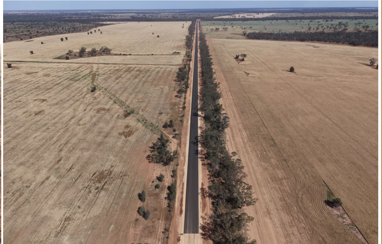
5km of 25km haul road completed and sealed
