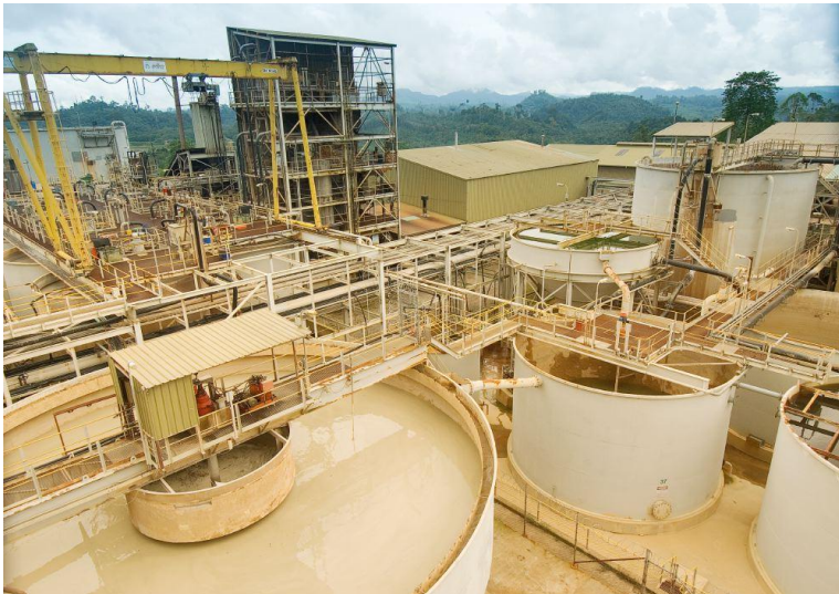
Mt Muro Leaching Circuit
