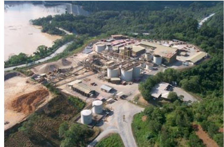
Mt Muro CIP / Merrill-Crowe Processing Plant
