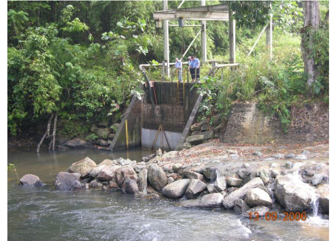
Menawing River Pumping Station
