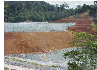
Sediment dam construction
