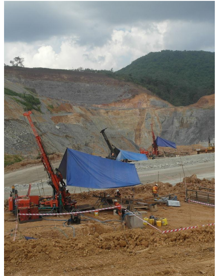
Diamond drilling, Permata resource drillout
