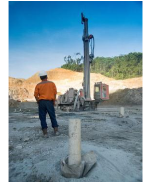
Drill and Blast
