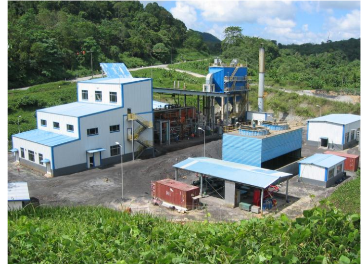
3.0 MW Coal Fired Power Station
