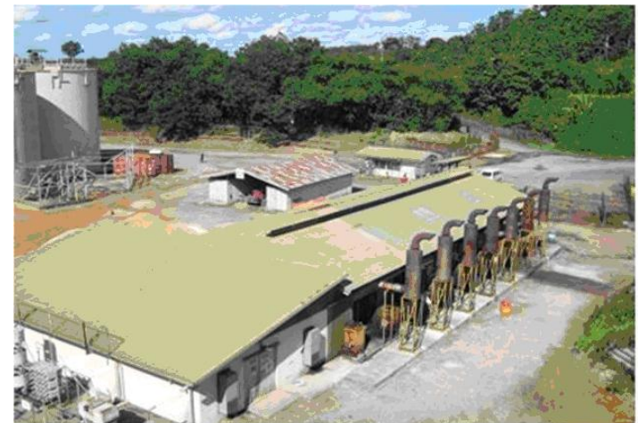
4.7 MW Diesel Power Station
