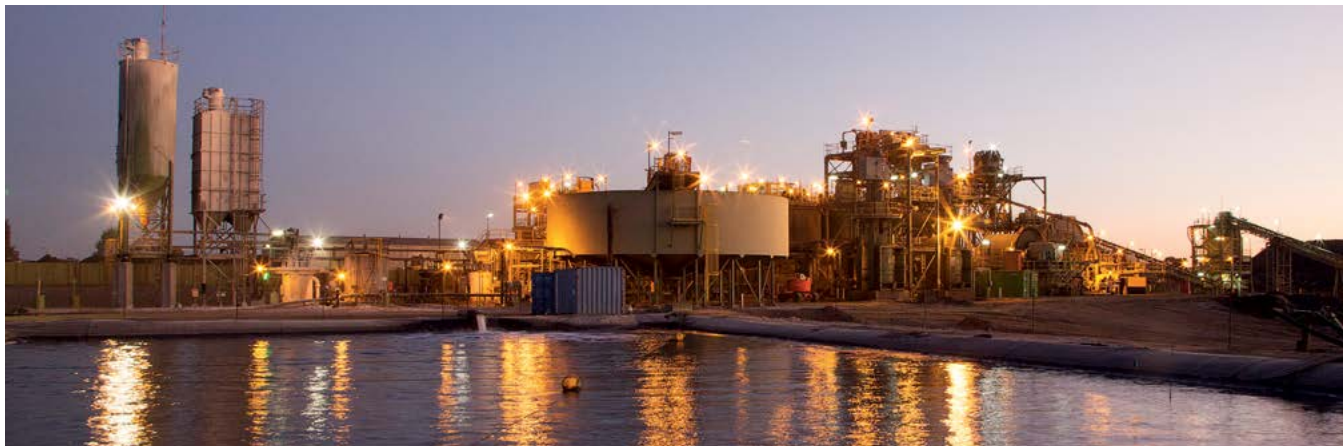
The processing plant at Straits' Tritton operations
