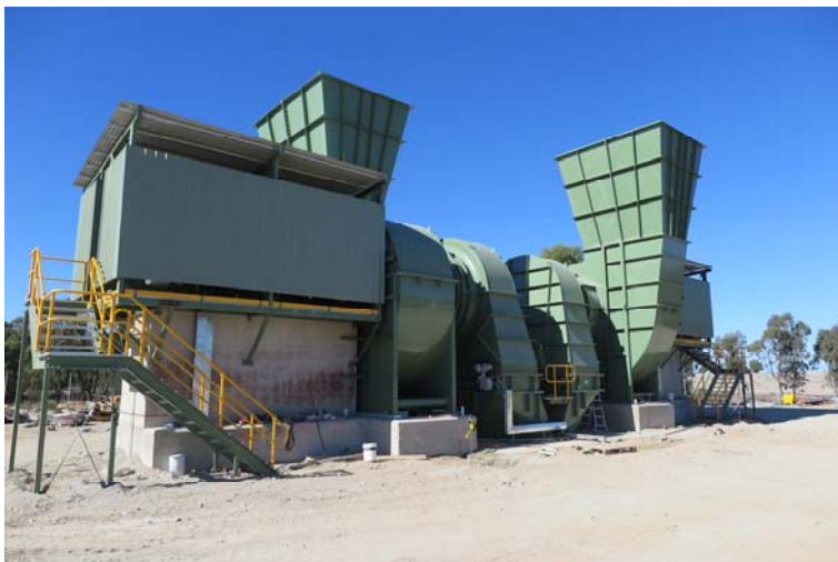
Figure 2: Ventilation Fans being installed at Tritton Underground Mine
