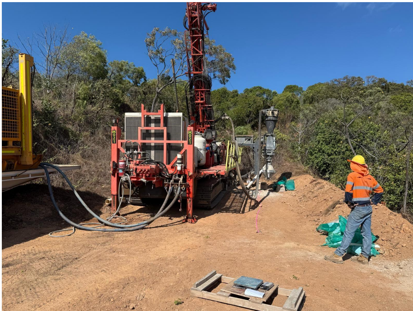
Figure 1. Drilling in progress at the Horn Island Gold Project.
