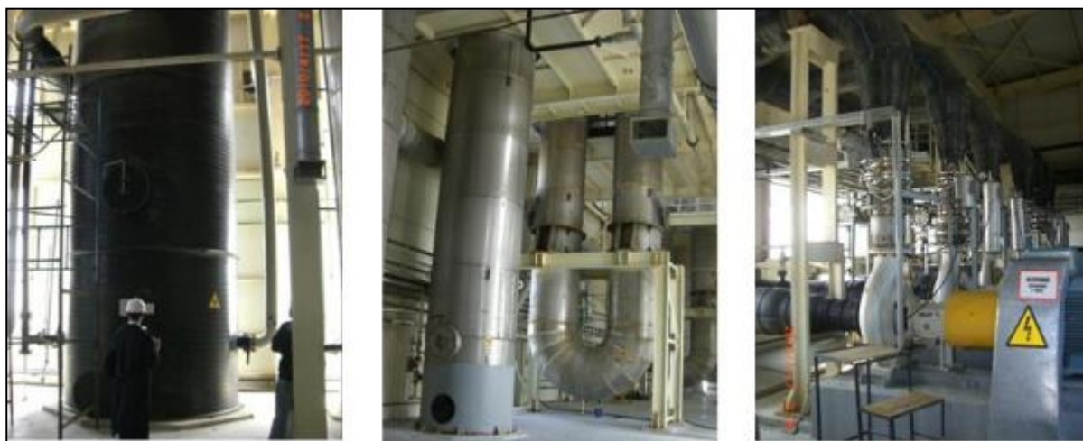
Figure 13-2: Continuous ion exchange plant with U-shaped columns in FSU (uranium)
