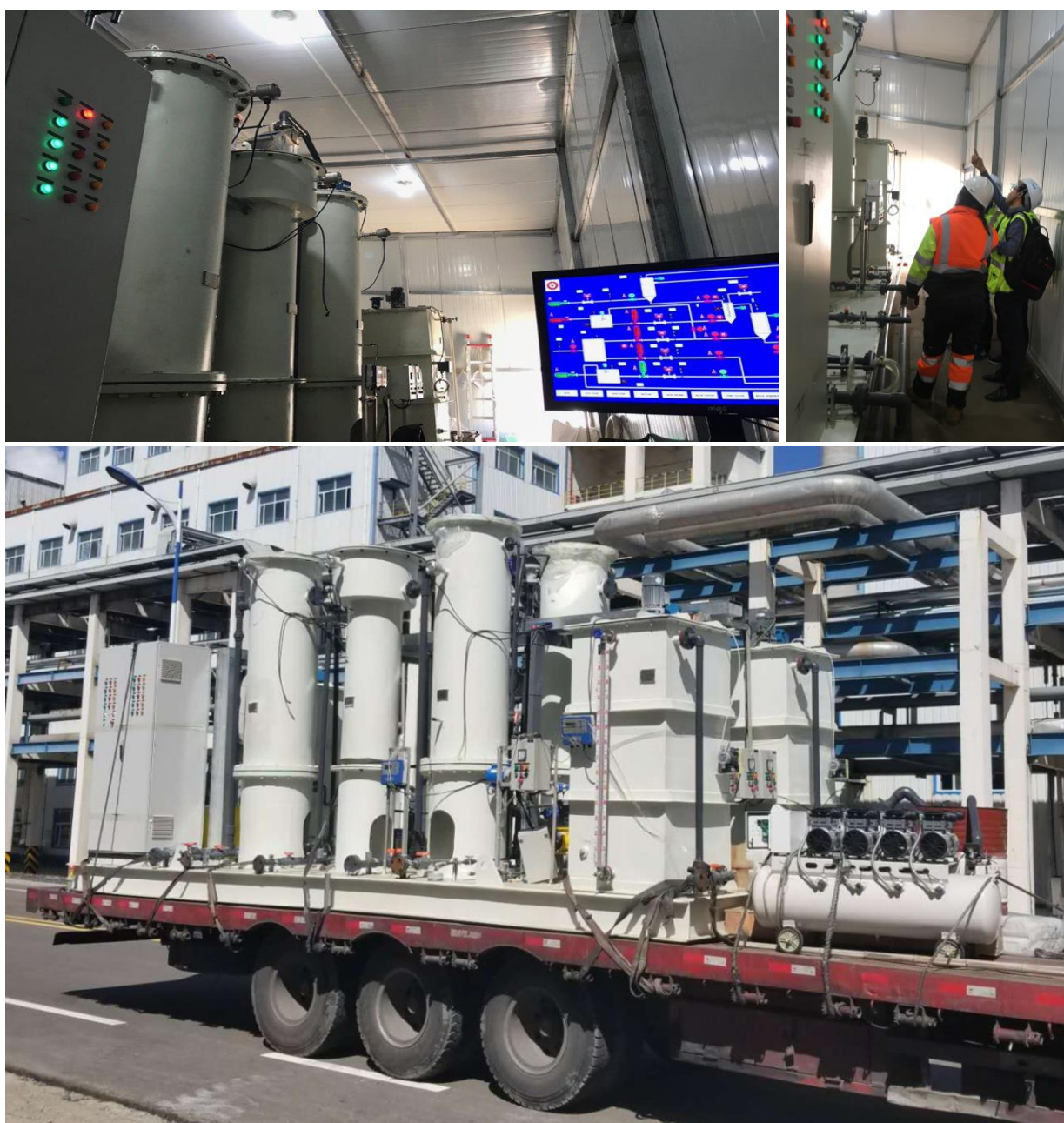
Figure 5 – Clean TeQ Continuous Ionic Filtration (CIF®) Mobile Demonstration Plant
