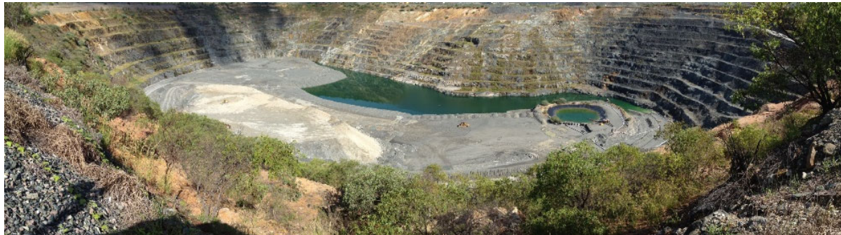
Pit 1 bulk backfill completed 17 August 2020
