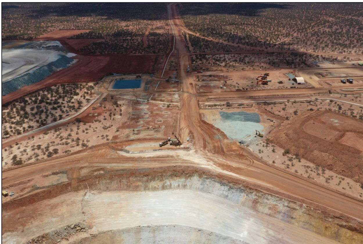
Figure 1: RC drilling currently in progress on the haul road running along the pit crest of the Gilbey’s Pit (view north).
