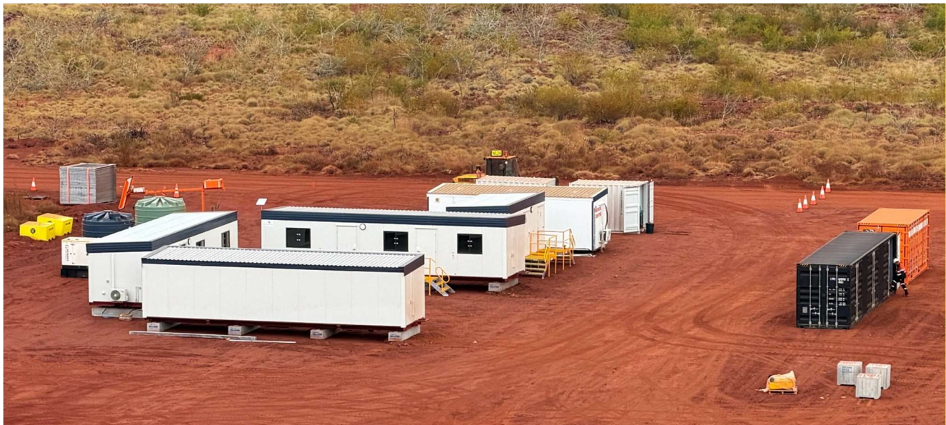
Figure 5 – BHP's NPI area established and constructed by Nyapiri Macro onsite at Mt Goldsworthy
