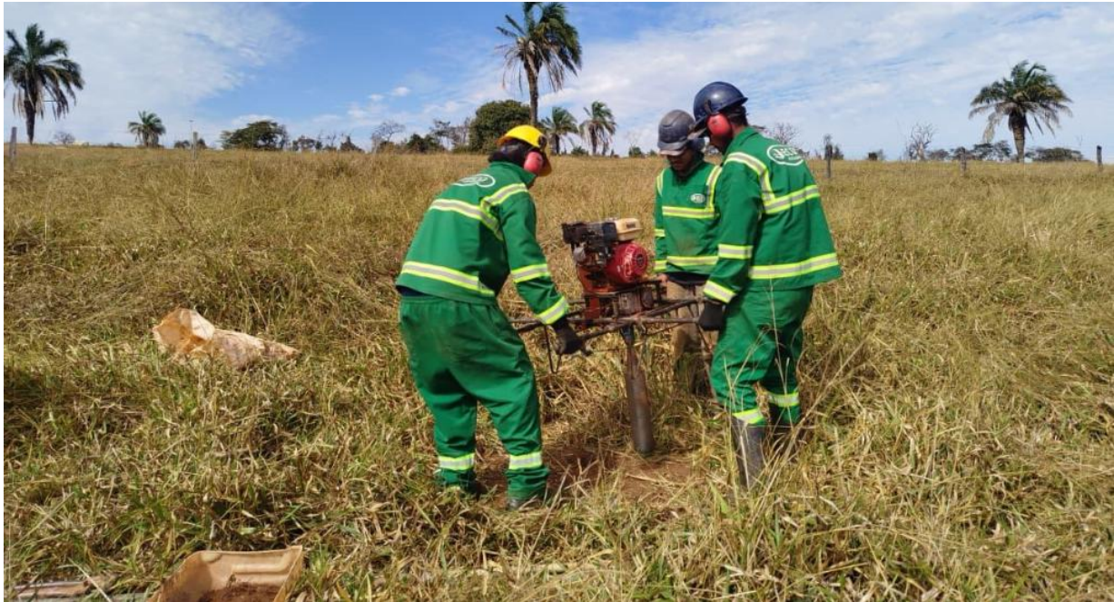
Figure 4: Drilling underway at Piracanjuba. Photo dated 30 June 2026.
