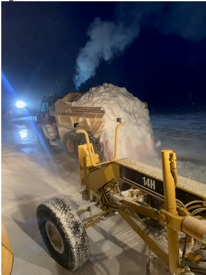
Fig. 1 Snow road construction
