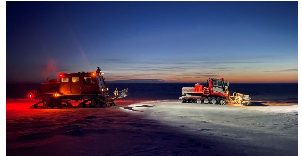
Commencement of snow road construction for Merlin-2
