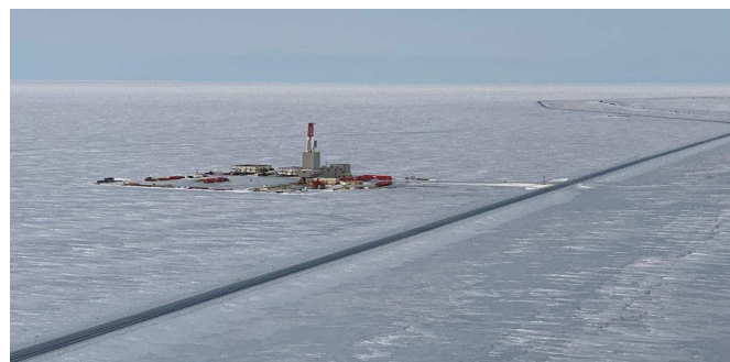
Figure 1: Project Phoenix' Hickory-1 well adjacent to Dalton Highway
