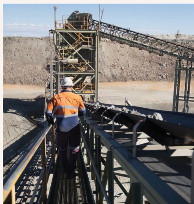
Tritton ore transfer conveyor
