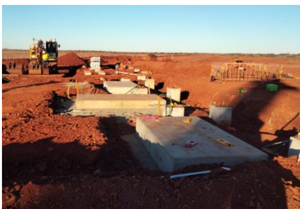
Figure 3: Transfer station 5/6 generator and switch room footings installation
