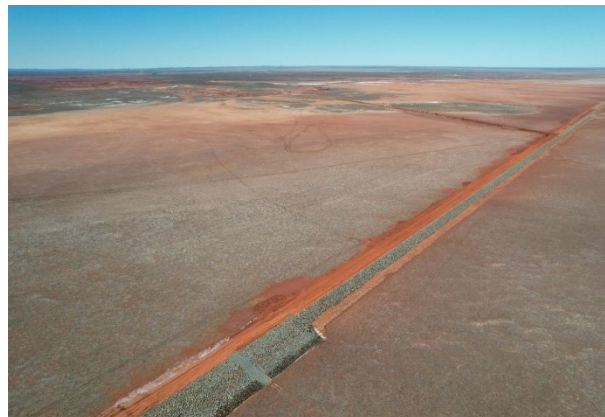
Figure 2: Pond 6 rock armour sea wall including spillway
