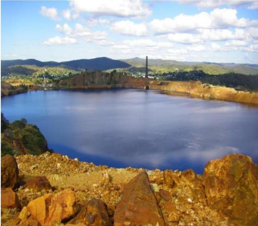
**Issue** | The tailings at the mine contains appreciable amounts of gold and copper. Conventional process routes for extraction of the gold are marginal. Furthermore, the legacy acid mine drainage problem needs to be solved concurrently with mine tails processing.
