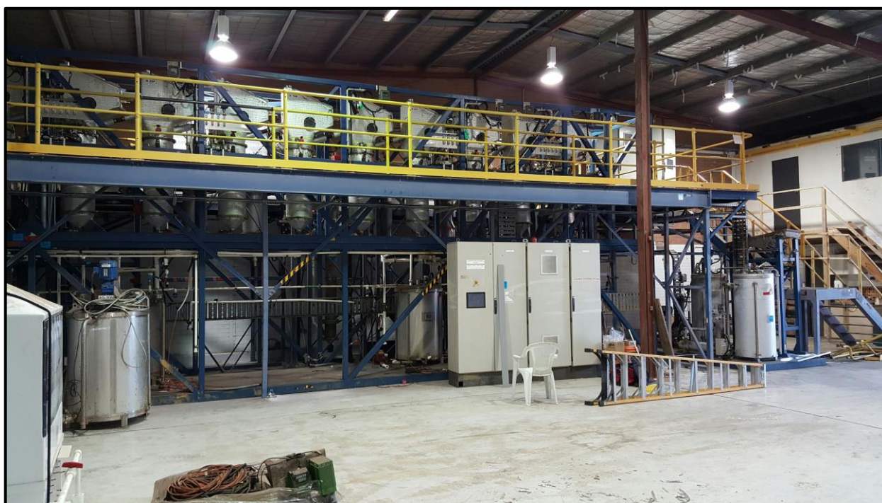
Clean TeQ's Resin-In-Pulp (RIP) pilot plant at ALS' facilities in Perth
