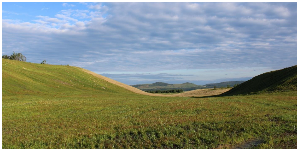
Completed rehabilitation at the Greenbrier mine.
