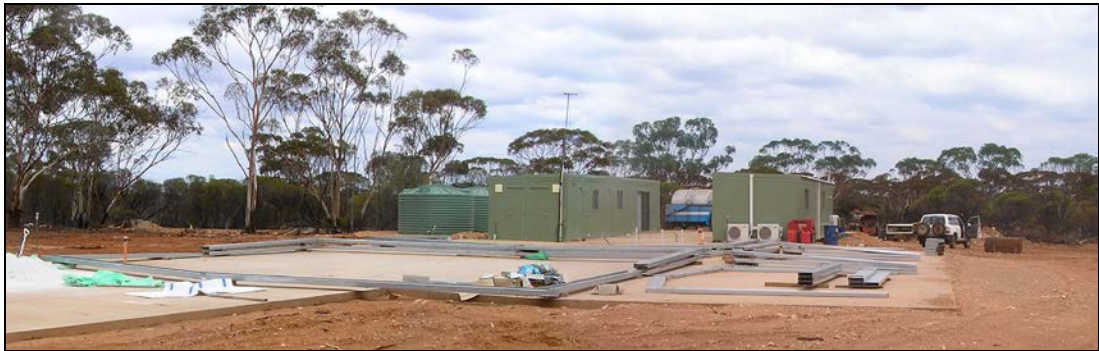
Figure 3 Administration Office Pad (foreground) Site Office/Cribs (rear)
