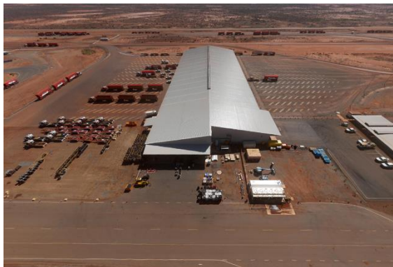
Truck maintenance facility
