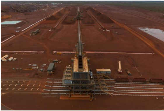
Truck loadout (TLO) facility
