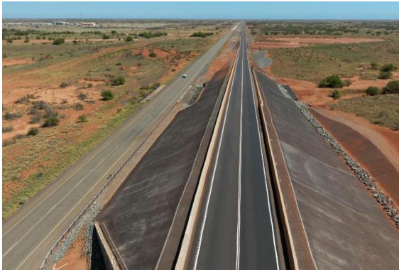
Upgraded section of Onslow Iron haul road
