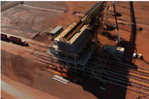
Road train loadout facility
