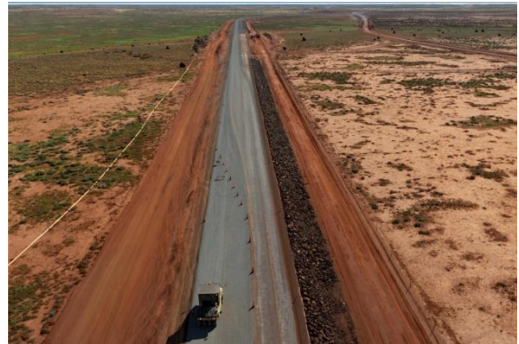
Haul road upgrade in progress
