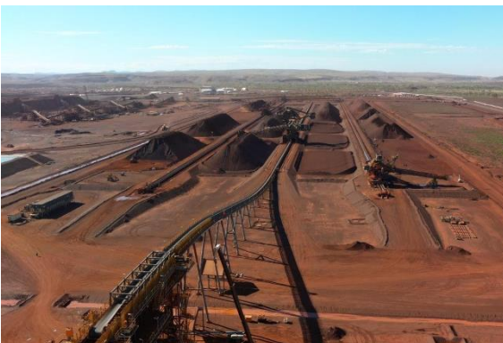
Ken's Bore stockyard
