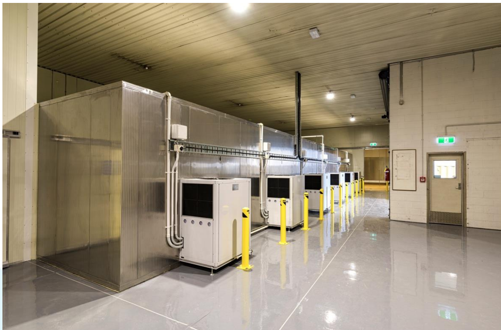
Image 1 – New Installed Driers shot from the Plant's General Circulation Area
